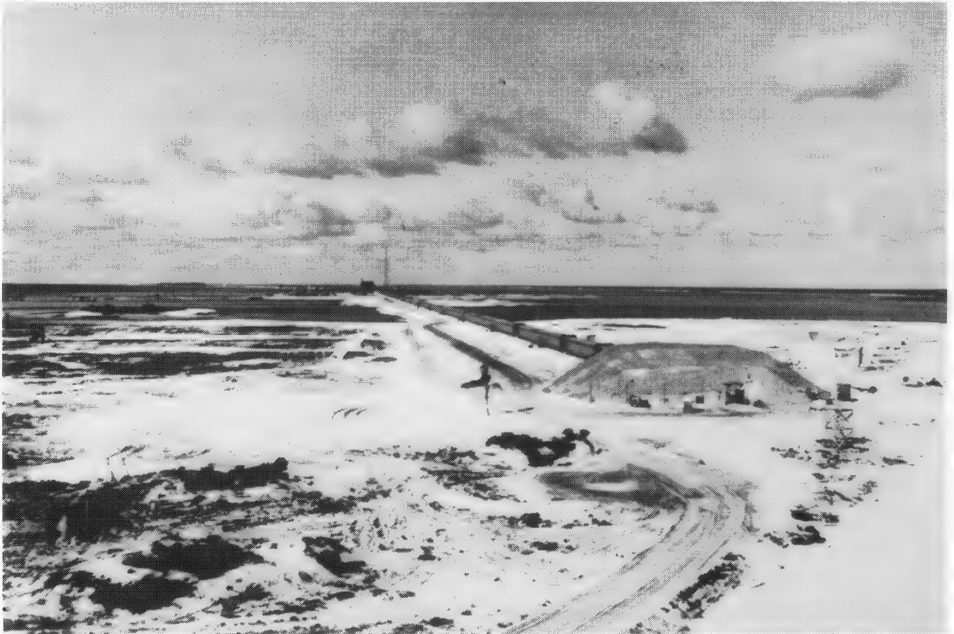
FIGURE 5-33. IVY MIKE D-1 (31 OCTOBER 1952) VIEWING NORTHWEST FROM STATION 200 TO SHOT CAB
