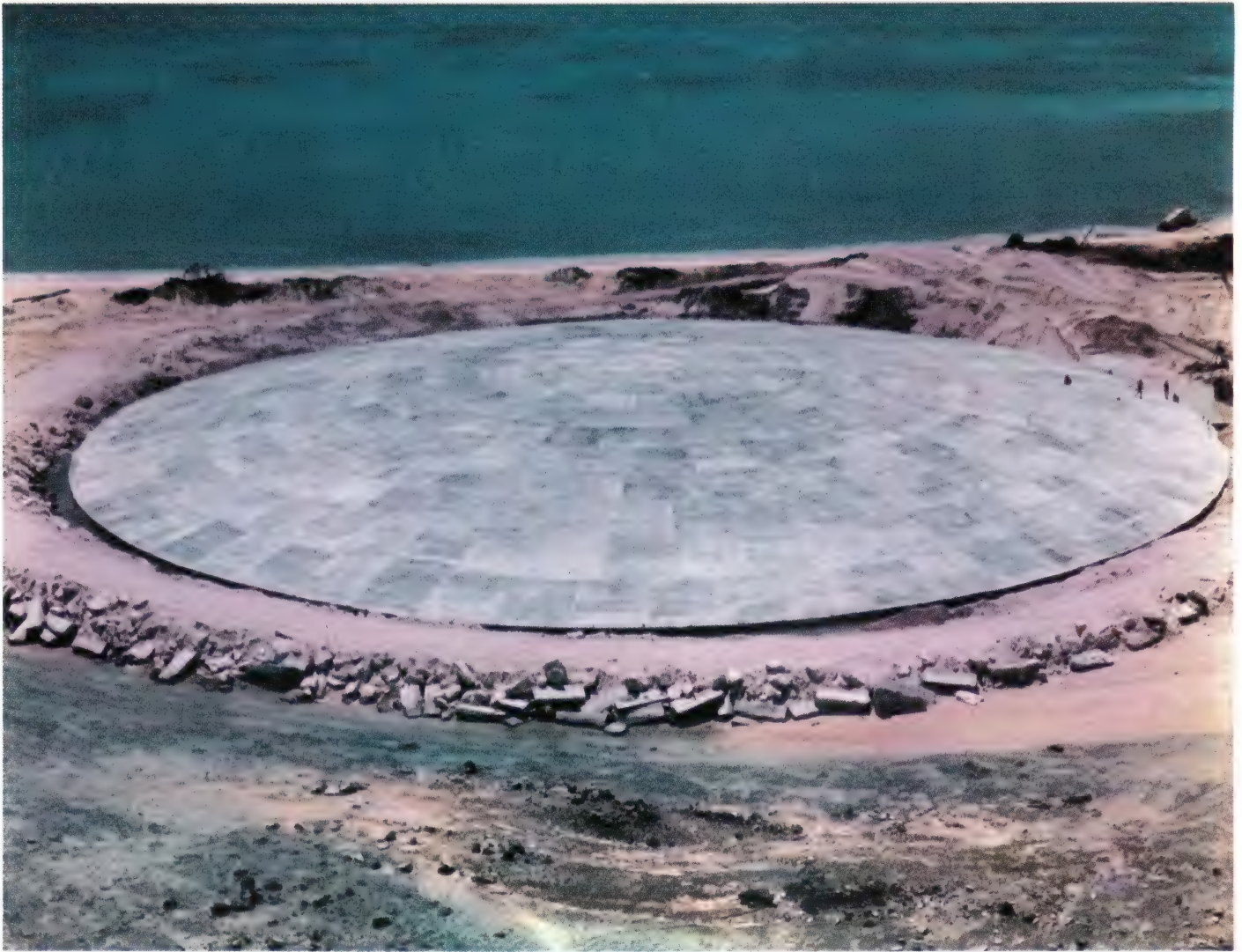
FIGURE 9-15. CACTUS DOME COVERS MOST NUCLEAR MATERIAL AT ENIWETOK ATOLL
