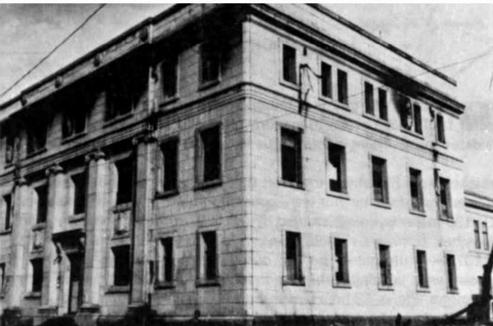
BANK OF JAPAN, HIROSHIMA (BUILDING 24)
