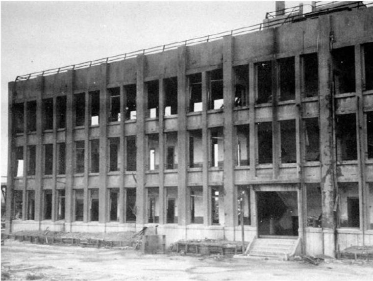
Above: 3-story concrete building 792 m west of ground zero Hiroshima. Firebrands entered through broken windows.
