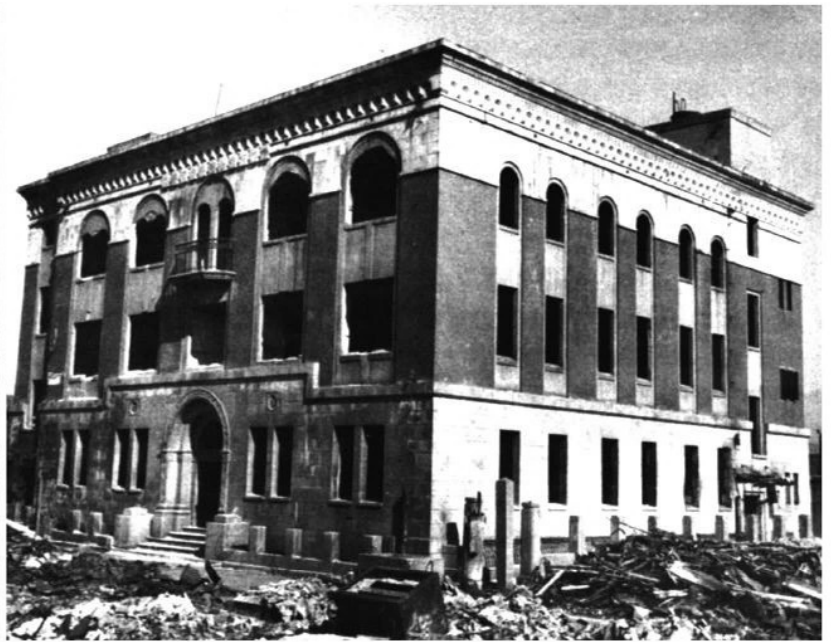
Above right: building 5, located at just 193 m from ground zero Hiroshima. Designed to survive a lateral load of 10% of its weight (Japanese minimal safety standard legislation).
