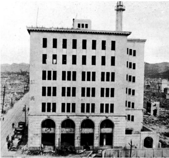
Above: building 18 (the 7-story Fukoku department store building), survived 20 psi peak overpressure blast at just 329 m from ground zero in Hiroshima. It burned hours later.
