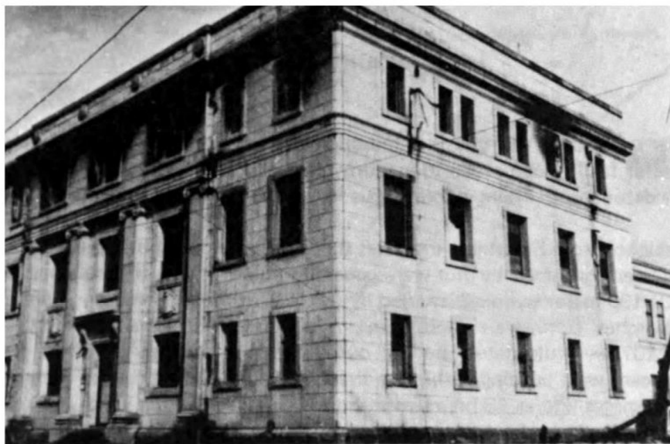
BANK OF JAPAN, HIROSHIMA (BUILDING 24)
