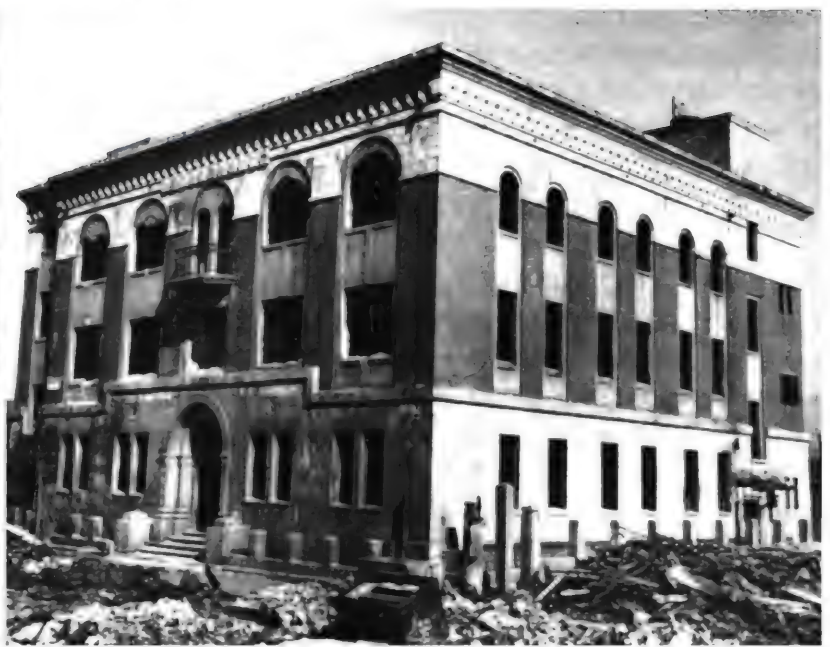
Above right: building 5, located at just 193 m from ground zero Hiroshima. Designed to survive a lateral load of 10% of its weight (Japanese minimal safety standard legislation).
