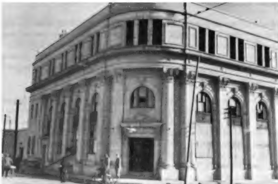
GEIBI BANK COMPANY, HIROSHIMA (BUILDING 18)
