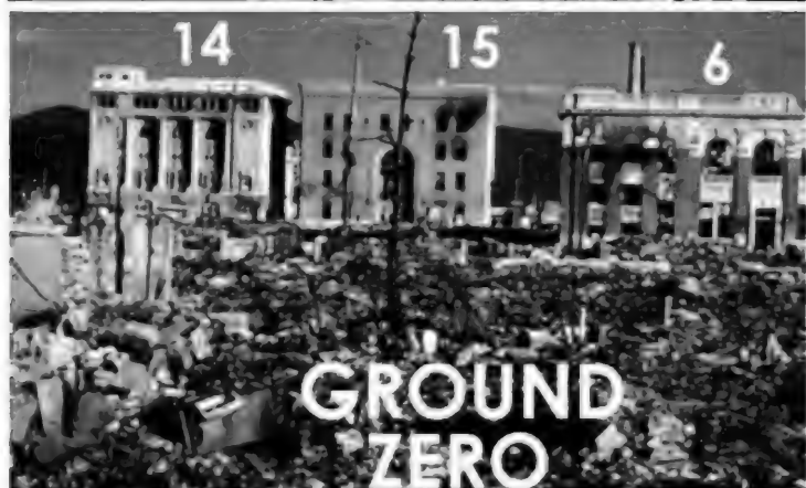
Above: U. S. Strategic Bombing Survey photos of Hiroshima. Even the closest bridge, south west from ground zero, remained service-
