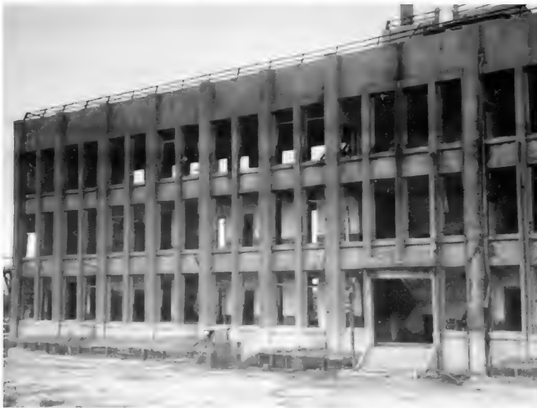
Above: 3-story concrete building 792 m west of ground zero Hiroshima. Firebrands entered through broken windows.
