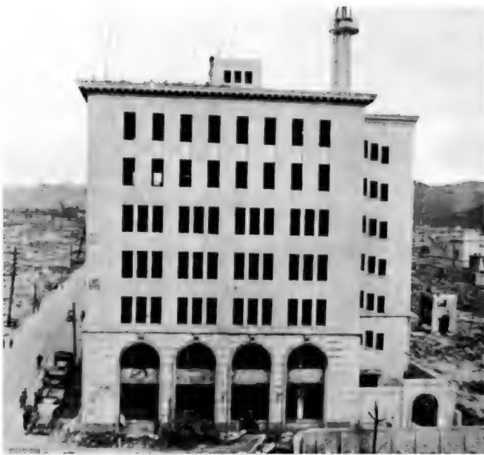
Above: building 18 (the 7-story Fukuoka department store building), survived 20 psi peak overpressure blast at just 329 m from ground zero in Hiroshima. It burned hours later.
