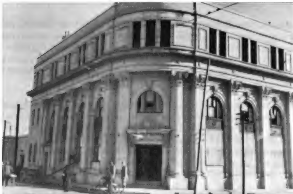
GEIBI BANK COMPANY, HIROSHIMA (BUILDING 18)
