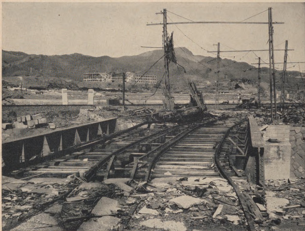
Figure 6.78. Steel plate girder railway bridge, about 280 yards from ground zero in Japan. The plate girders were moved about 3 feet by the blast, but the bridge was essentially intact.
