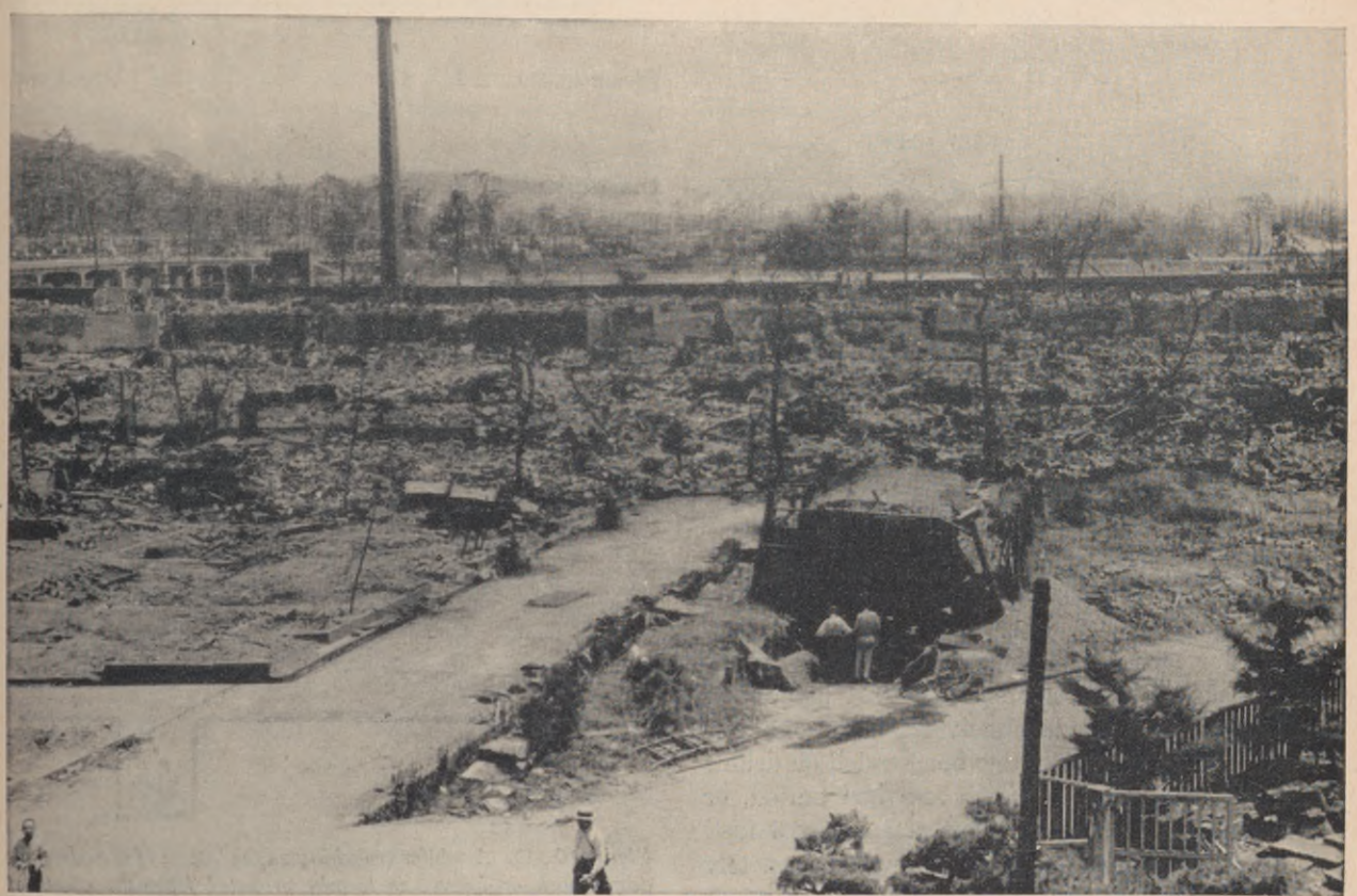
Figure 10.39. Simple pole and earth shelter, one mile from ground zero, undamaged by fire and blast although surrounding buildings were destroyed in the atomic bombing of Japan. (Debris was cleared from the roadways before the photograph was taken.)
