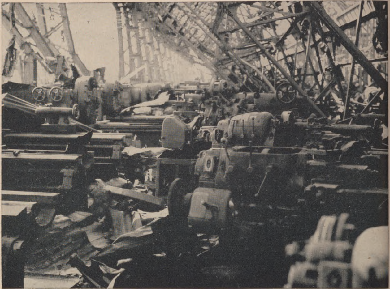
Figure 6.84. Machinery lightly damaged by debris and by fire, but exposed to the elements after the atomic attack on Japan.
