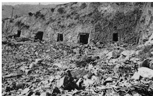
Figure 12.52a. Tunnel shelters in hillside, very close to ground zero in Nagasaki, protected the occupants from blast and from thermal and nuclear radiations.
