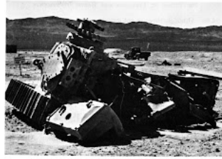
Figure 12.4k: Earth-moving equipment subjected to nuclear blast in open terrain (30 psi overpressure).
