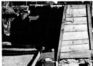
Figure 12.27c. Earth-filled, wooden blast walls protecting machinery (0.85 mile from ground zero at Nagasaki).
