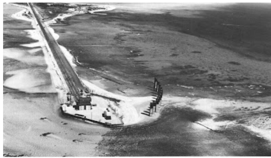
Station 22. "Castle Bravo" shot site at end of 2,000 ft. runway westward of Huru Island, Bikini Atoll, January 1954. The 7,500 ft. 12-pipe diagnostic array stretches into the background. Semicyclic air of reflecting mirror covers (Station 1355.1) through 1350.12 stands to right of shot cas. Mirror reflected early burst explosion light to "swamp" beneath a low ridge slope. (LANL, 2-15-54)
