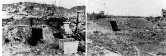
Fig. D.1. A small, earth-covered backyard shelter with a crude wooden frame—undamaged, although only 300 yards from ground zero at Hiroshima.
