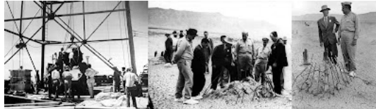
Above: even with a relatively heavy design and casing (thus maximum cratering action relative to modern lighter weapons of comparable yield), the TRINITY (19 kt, 30 m altitude, 16 July 1945) test left the foundations of the steel tower behind in the middle of the crater, as photographed on 11 September 1945. A wide shallow crater was scoured out by the shock wave, but hardened underground structures could have survived, which is why surface bursts are required to destroy such targets.
