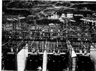
Figure 12.27b. Reinforced-concrete blast walls protecting transformers (1 mile from ground zero at Nagasaki).
