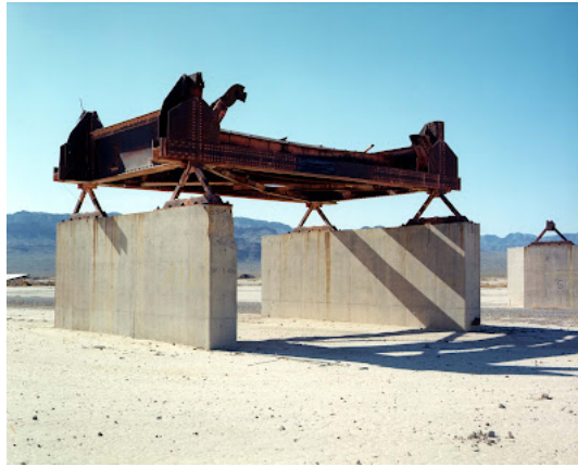
Above: This railroad bridge segment at 1,800 feet from the 37 kt PRISCILLA Nevada test in 1957 survived a peak overpressure of 450 psi but had severe distorting to its internal structure.
